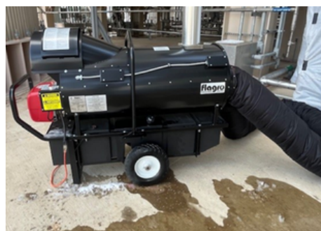
Portable industrial heater to warm temporary enclosure
