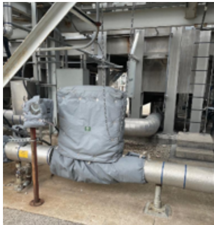
Custom-fit insulation covers to protect irregular shaped and hard-to-reach components
