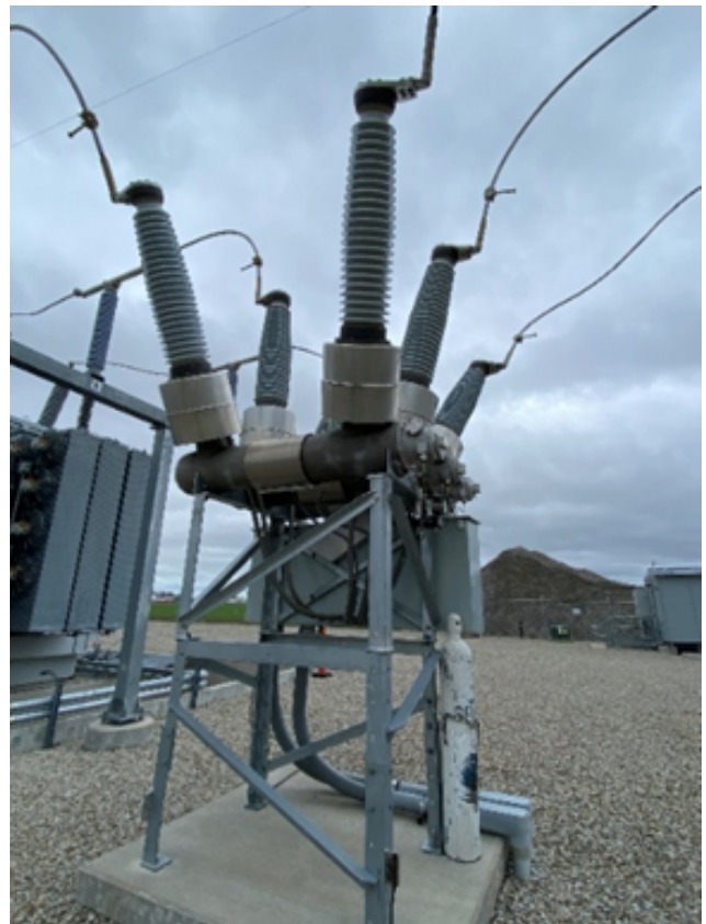
Typical SF6 breakers installed at an IBR
