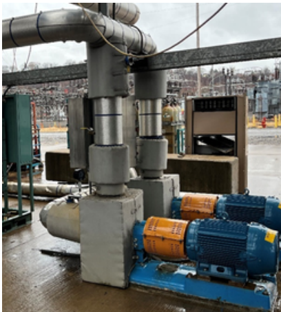
Custom-fit insulation covers to protect irregular shaped and hard-to-reach components
