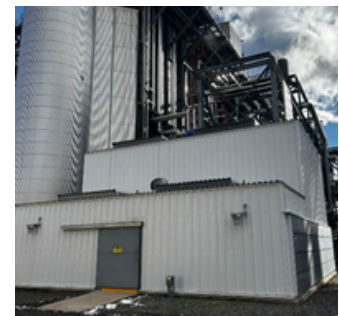
Main turbine building protects most critical components from freezing
