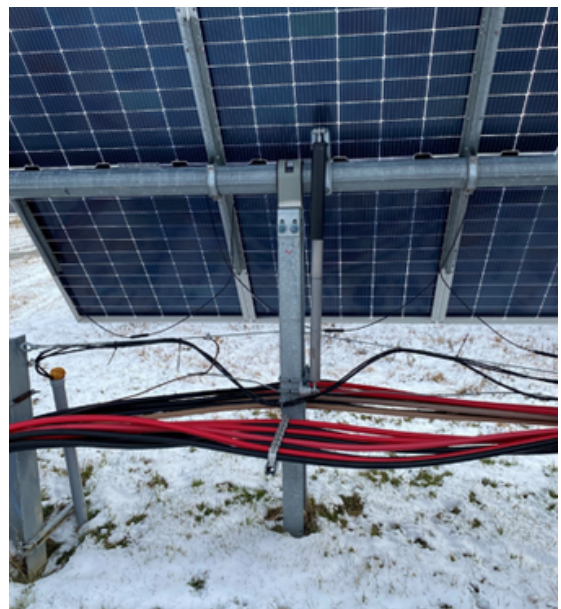
Bifacial solar panels, which draw power from both front and rear
