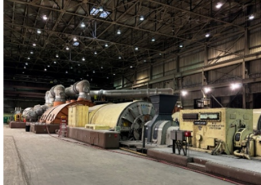
Main turbine building protects most critical components from freezing
