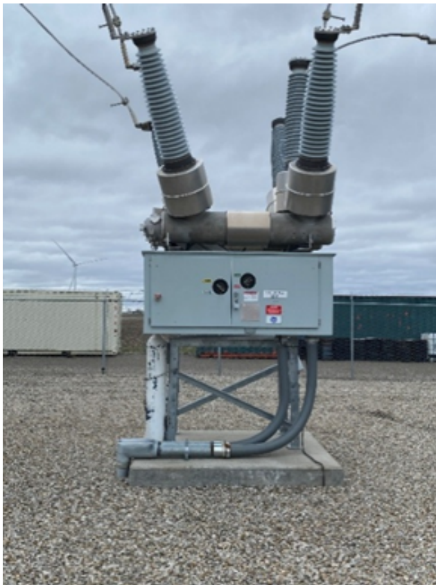
Typical SF6 breakers installed at an IBR
