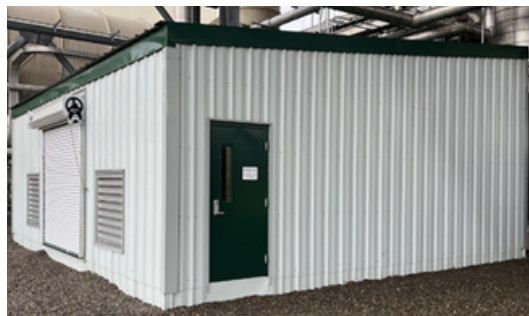
Main turbine building protects most critical components from freezing
