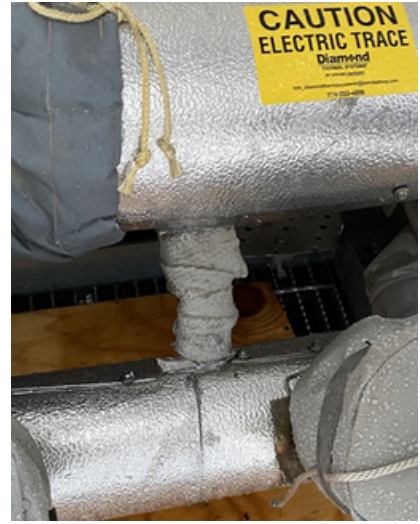
Insulation of structural support between piping to reduce heat transfer
