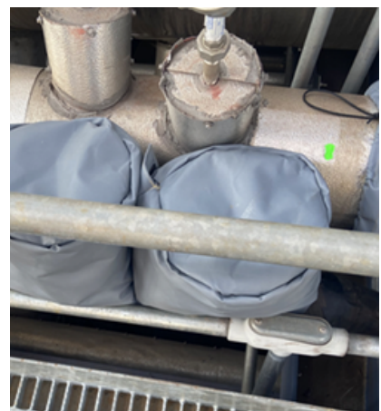
Custom-fit insulation covers to protect irregular shaped and hard-to-reach components
