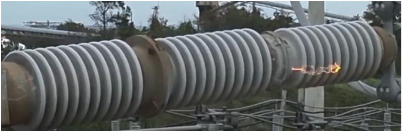
Figure 3: Brandon Shores 230 kV insulator with tracking
