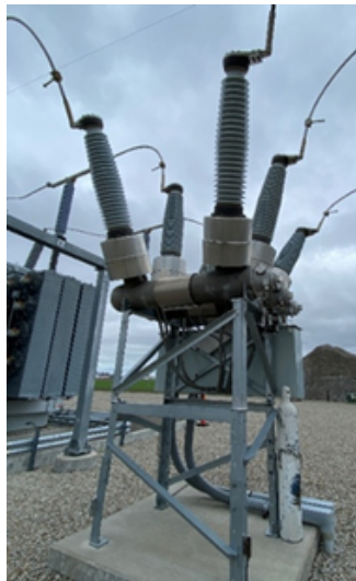
Above: Typical SF6 breakers installed at an IBR.
