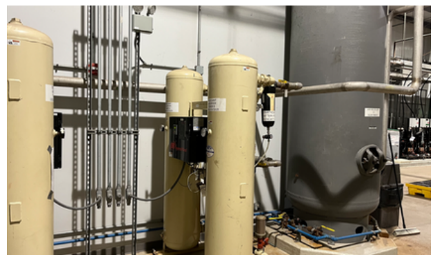
Compressed air supply system
