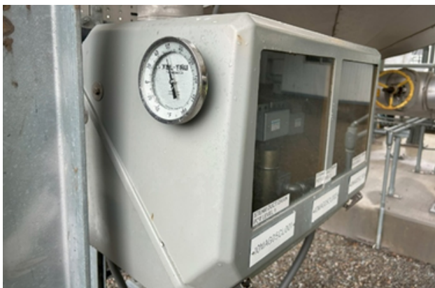
Above: Local visual temperature indication on transmitter enclosures.
