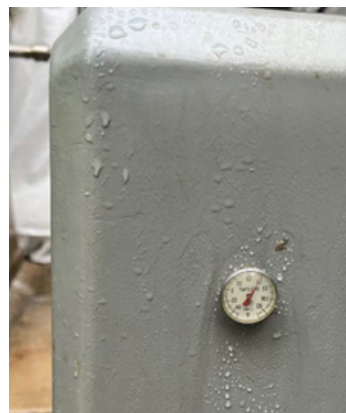
Above: Local visual temperature indication on transmitter enclosures.
