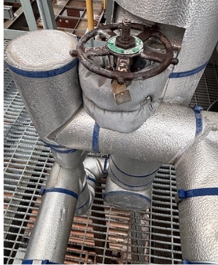
Valve stem with insulation
