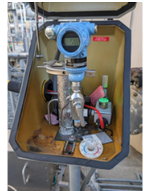
Above: This entity uses an indicating light and a small thermometer in the transmitter enclosure box to assist operators during inspection rounds helping to demonstrate proper heater functioning.
