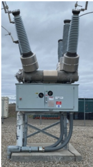
Above: Typical SF6 breakers installed at an IBR.
