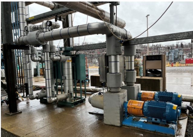
Custom-fit insulation covers to protect irregular shaped and hard-to-reach components
