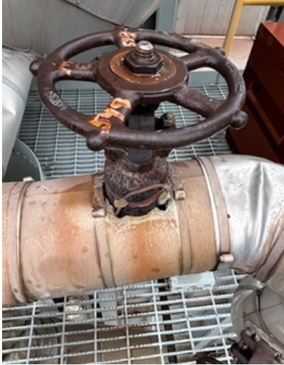
Valve stem without insulation
