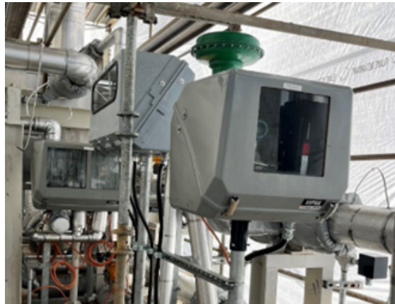
Left: Transmitter manifold assembly enclosed by a protective clamshell using an internal heater.
