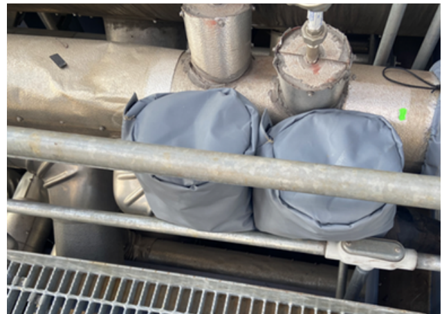
Custom-fit insulation covers to protect irregular shaped and hard-to-reach components
