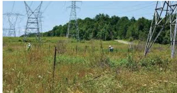
*Photo: Electrical Contractor Magazine
