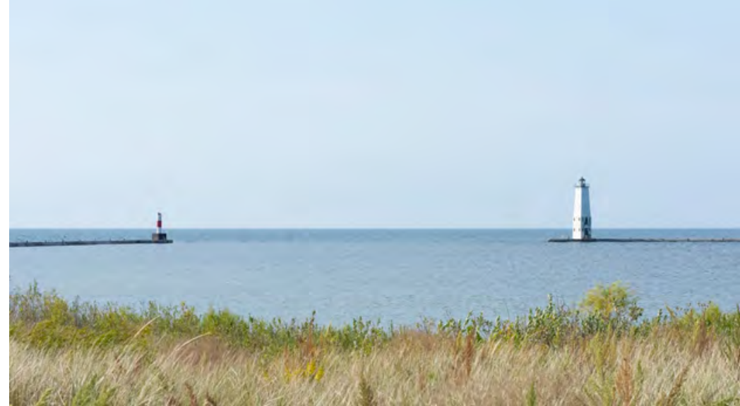
Frankfort South and North Breakwater, MI – Photo: L Folkerth
