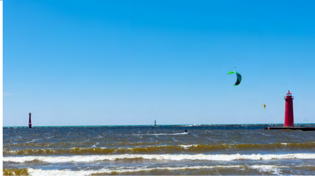
Muskegon, MI: S & N Breakwater, S Pier – Photo: L Folkerth
